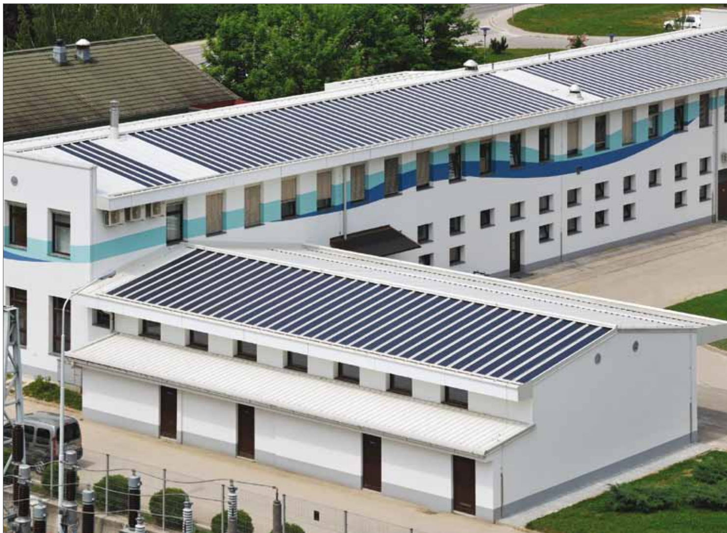
FIG. 14: RATED POWER OF THE PV POWER PLANT: 38,08 kWp
