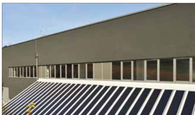
FIG. 16: RATED POWER OF THE PV POWER PLANT: 4,08 kWp
